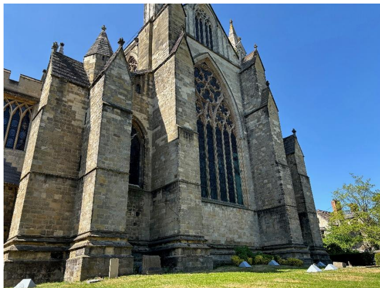
Figure 4: East end of church. Note the strong buttressing
